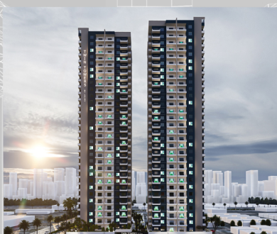
LALAV TWIN TOWERS
